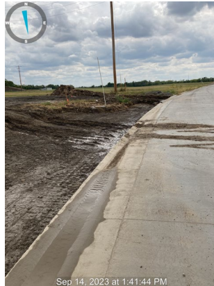
2. Track out of sediment was seen at several residential construction sites.
