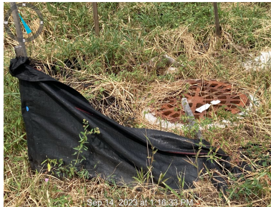
2. Riverdell- Inlet silt fence BMP has not been maintained.
