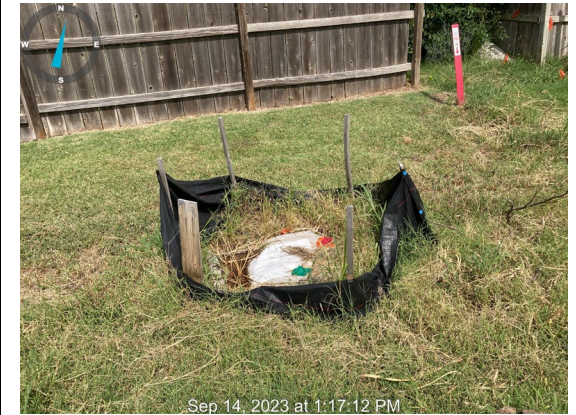
3. Riverdell- Another inlet silt fence that has been maintained.
