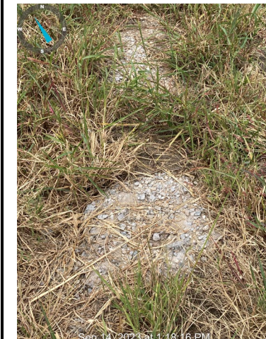
6. Riverdell- Concrete washouts on the ground. No washout containment on site.
