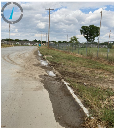
1. No back of curb protection allowed dirt to seep out to the street.
