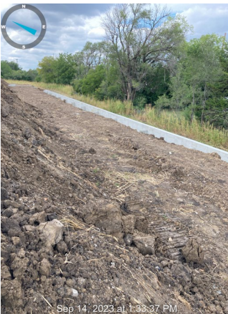
5. Retaining wall to hold back sediment on the backside of this mound.
